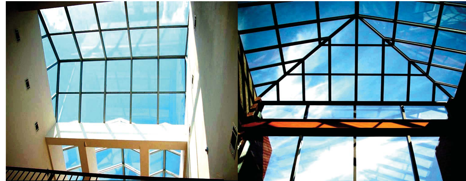
COMMERCIAL BUILDING Profile: Double Pitch Ridge with Gable End Location: Brooklyn, NY
